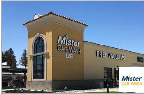
Mister Car Wash Orlando, FL
